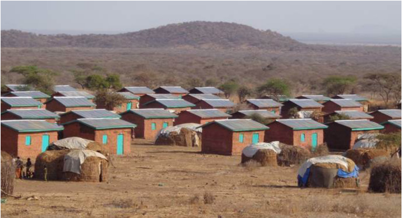
Improved transitional shelter constructed for Kenyan Borena refugees in Megado and Dillo camps. (UNHCR Support)
