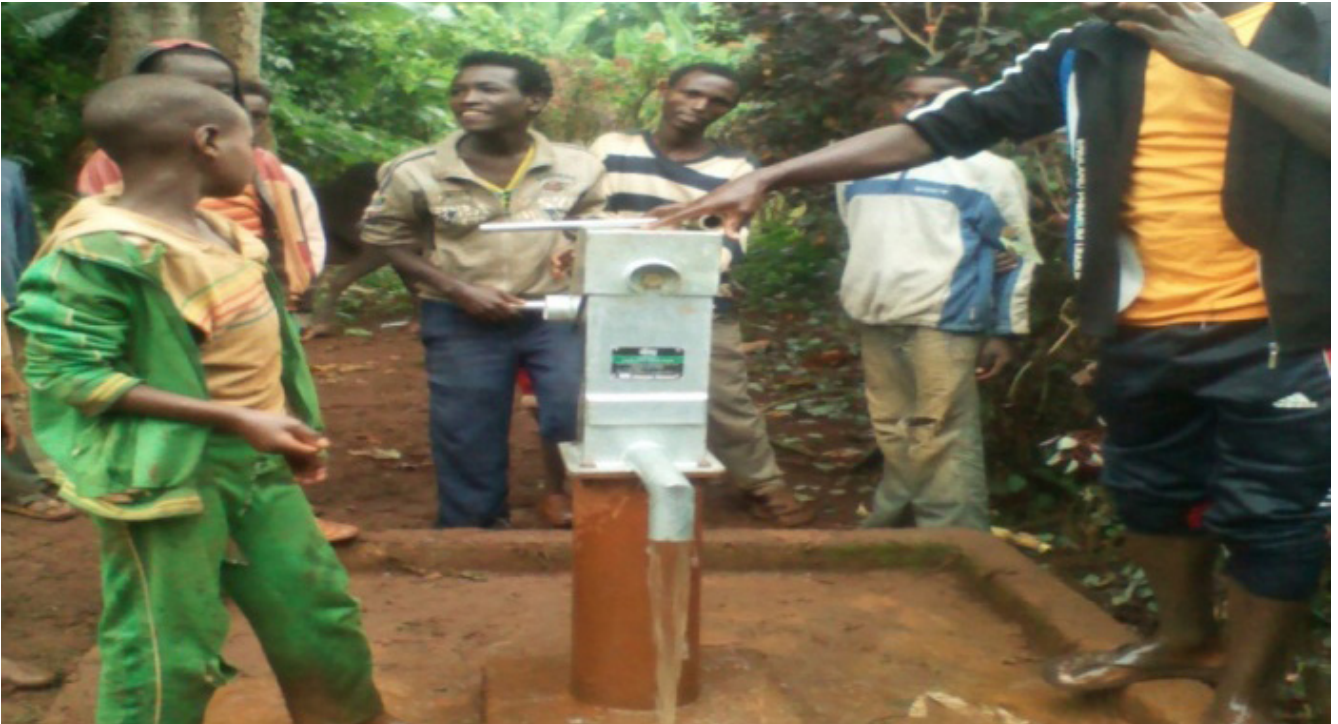
Rehabilitation of water schemes at Bule-Hora Woreda (TIKA Support)
