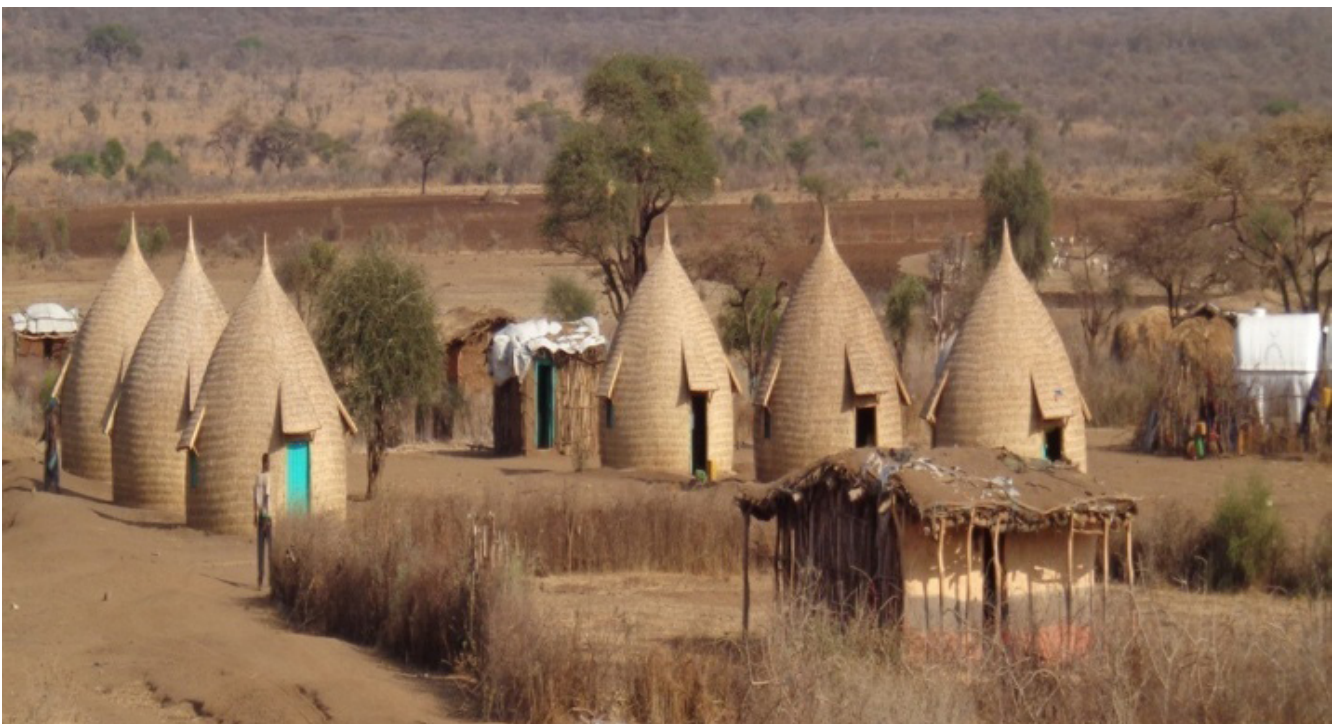
Improved transitional shelter constructed for Kenyan Borena refugees in Megado and Dillo camps. (UNHCR Support)
