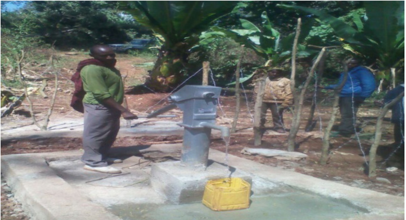
Rural water development project in Bule Hora woreda of Borena zone (Japan Embassy Support)
