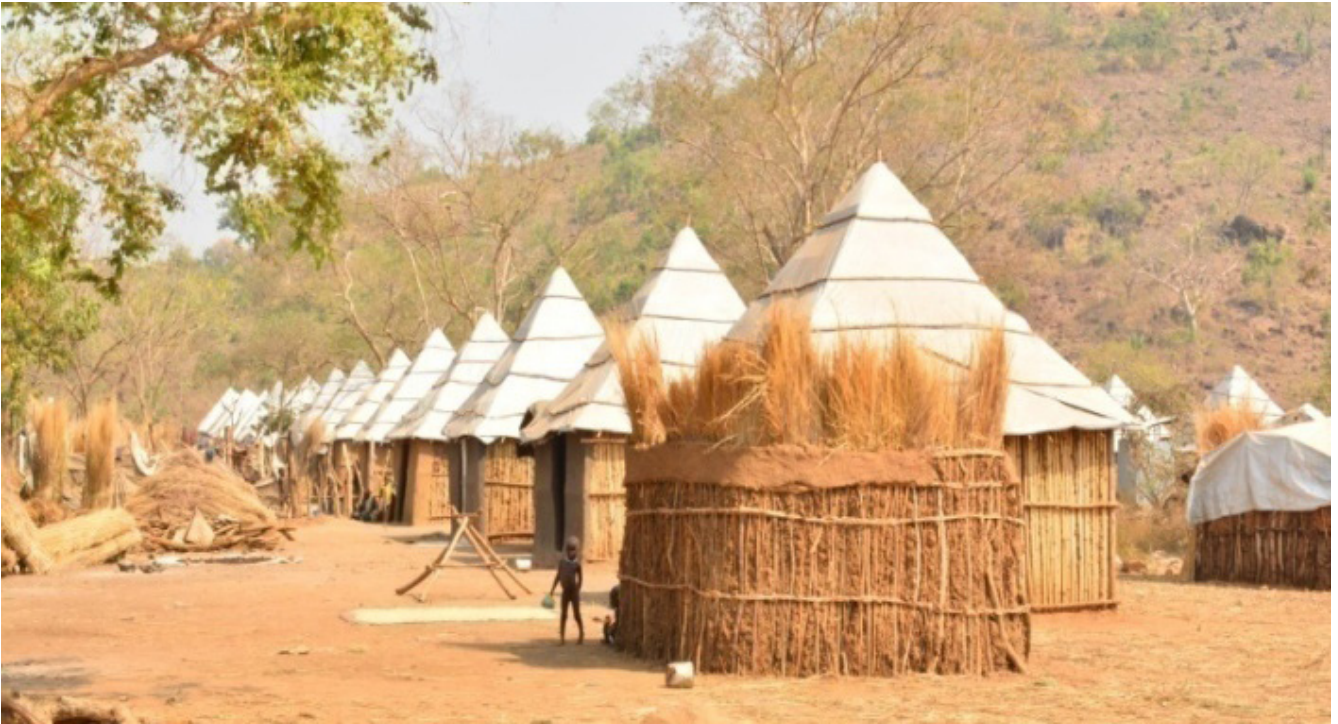
Transitional shelter constructed for south Sudanese refugee in Terkidi refugee camp Gambella (UNHCR Support)
